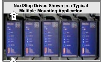
NextStep Drives Shown in a Typical Multiple-Mounting Application
