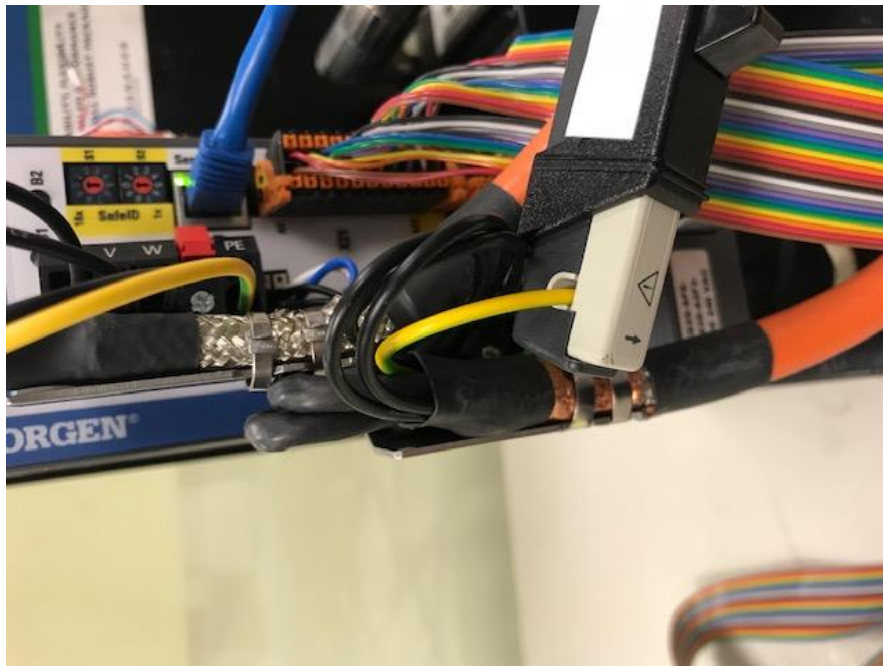
Figure 11: Using a current probe to monitor the safety ground.
