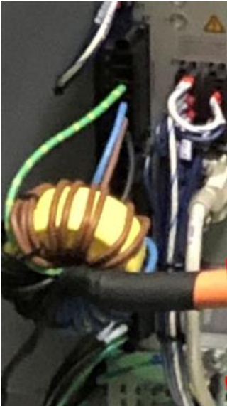
Figure 19: Common mode custom inductor created with the Micrometals powdered iron cores. These or other cores are commonly used for HF noise on the shield caused by common mode noise creating stray currents on the long cables and transmitting magnetically into the surrounding systems.
